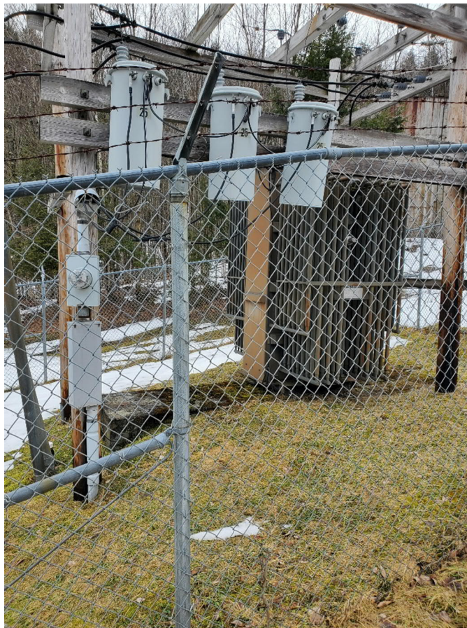
Photograph #2: Existing Transformer and Bus Structure
