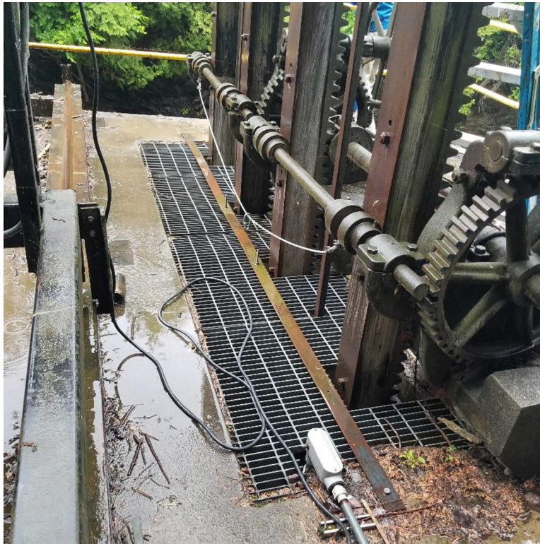
Photograph #3: Existing Headgate Support Arms and Actuators
