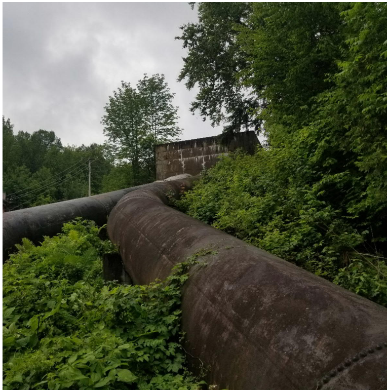
Photograph #4: Existing Unit No.2 Penstock
