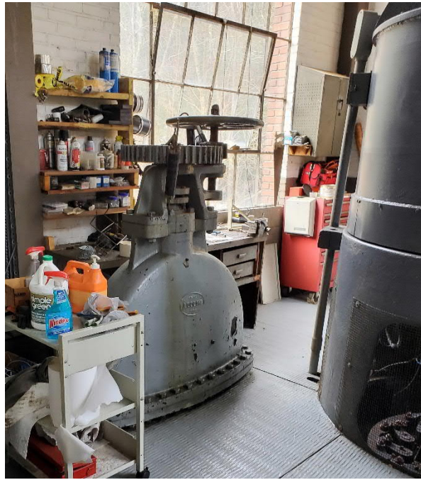
Photograph #1: Existing Unit No.2 Penstock gate Valve
